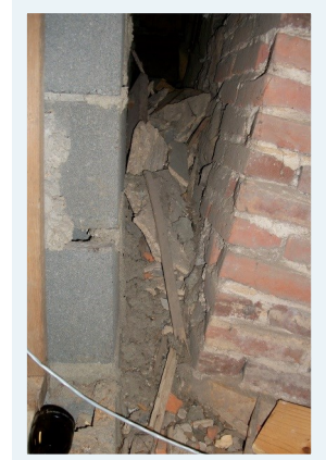
Brick wall leaned out behind CMU wall
