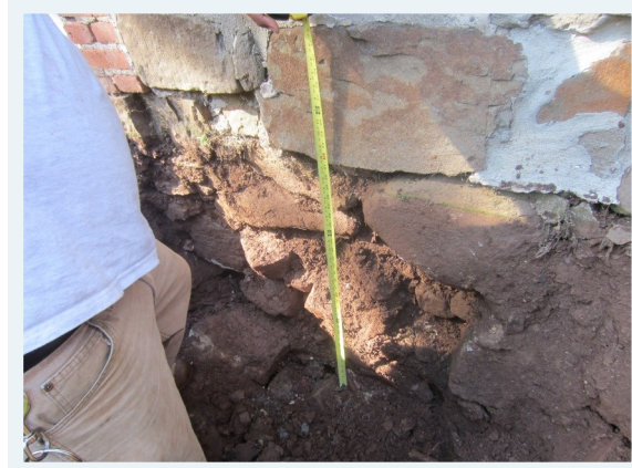
Exterior probe showed bottom of fieldstone wall sat on dirt at the frost line
