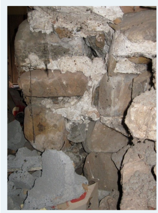
Fieldstone foundation at north wall had collapsed
